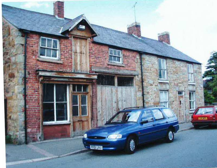
Old Butcher's Shop, Northop BLI before restoration
