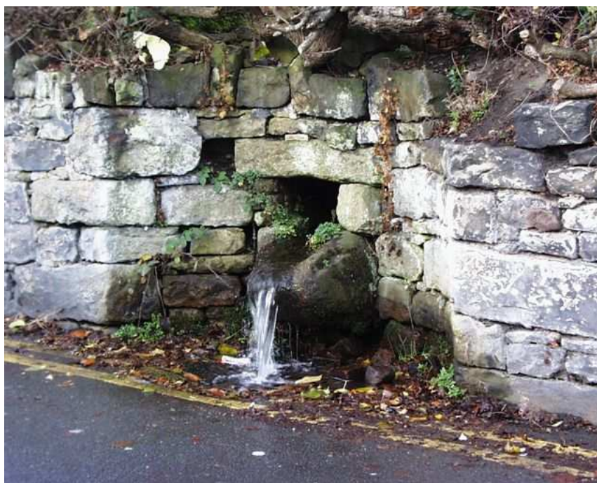
BLI structure - Pistyll in Caergwrle
